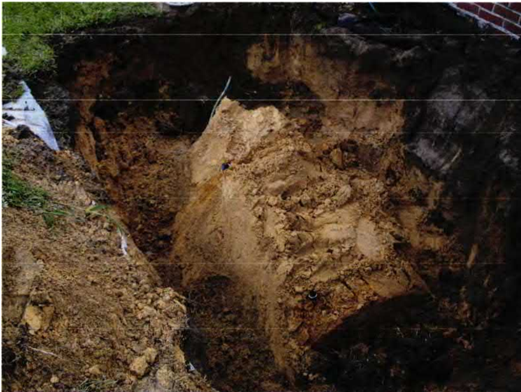
Picture 2: UST 1257Dove shortly before removal.
